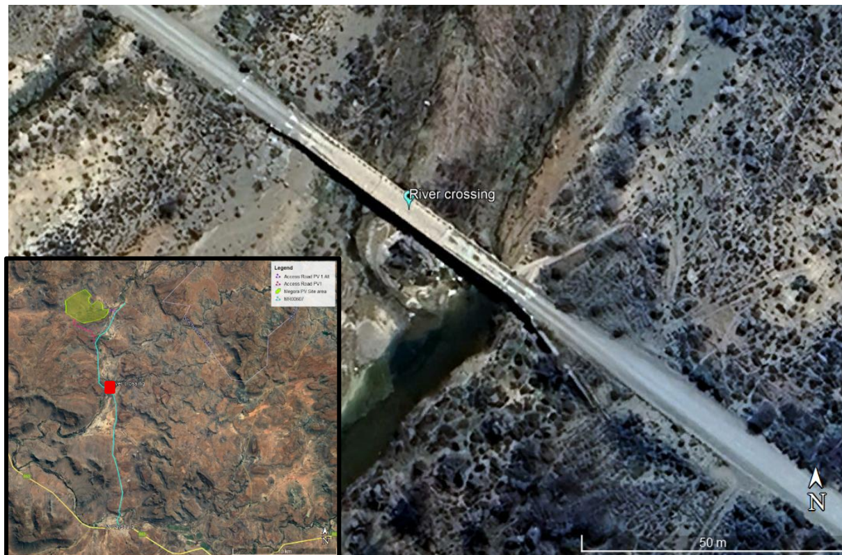
Figure B.7: Aerial View of Bridge located on MR00607 (Source: iWink, 2025)
