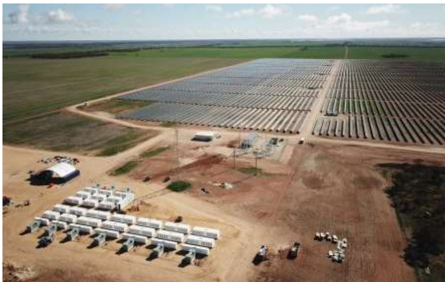
Figure 2.5: Example of PV Technology with Lithium-Ion BESS in the foreground (ARENAWIRE, 2018 2 )
